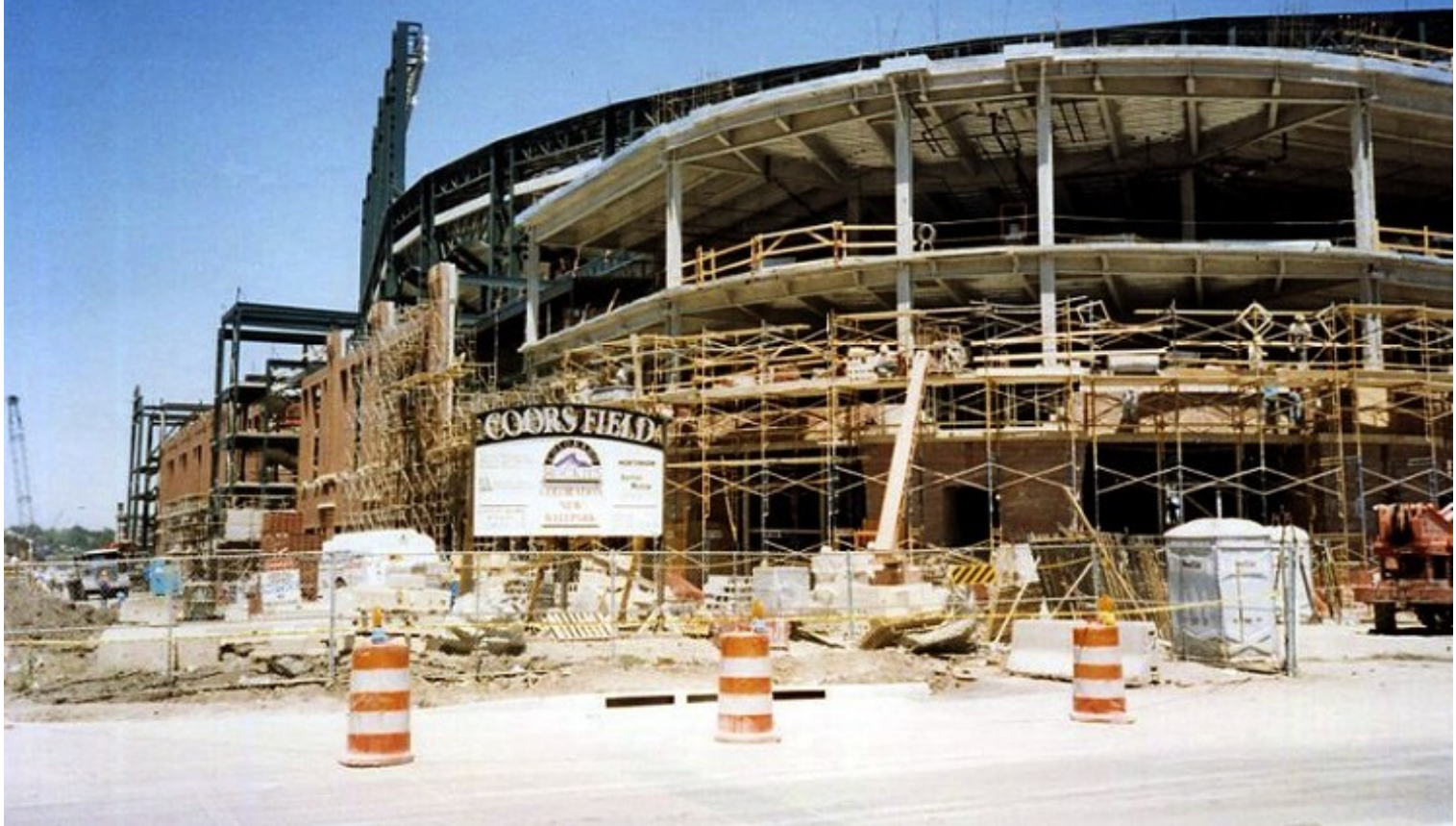
Coors Field under construction in 1994. / Jonathan Shikes
